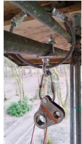
All safety ropes pass over a sheer reduction block.
