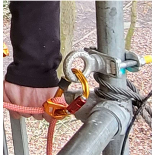
Instructor using a Petzl Connect personal anchor on one of the corner anchor rings.
